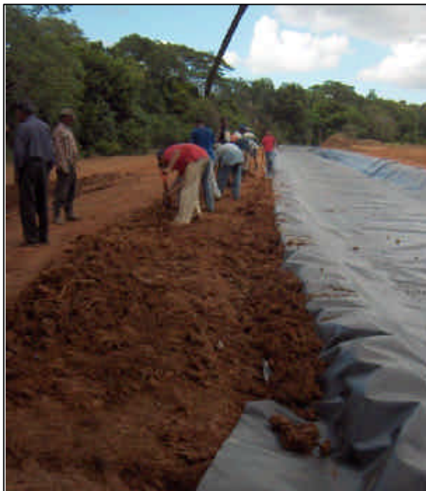
Construction of a Filter with macrophytes floating in Dominican Republic (November 2005).
